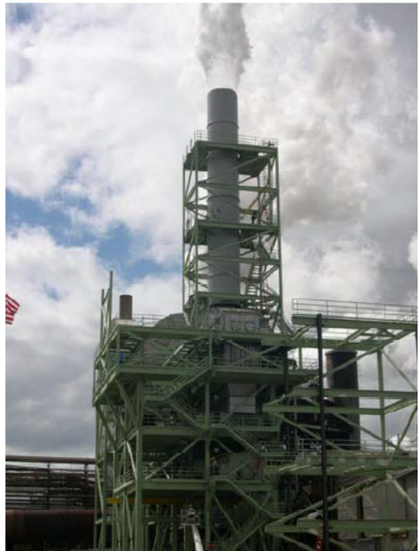
Wet ESP on Power Boiler
