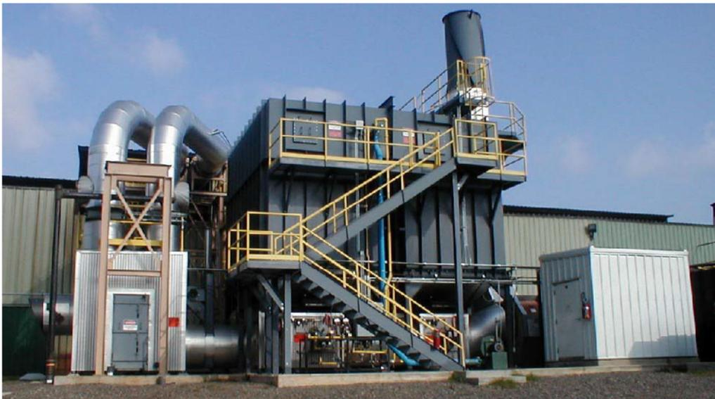
Regenerative catalytic oxidizer on a veneer dryer at Weyerhaeuser plant in Zwolle, La.
