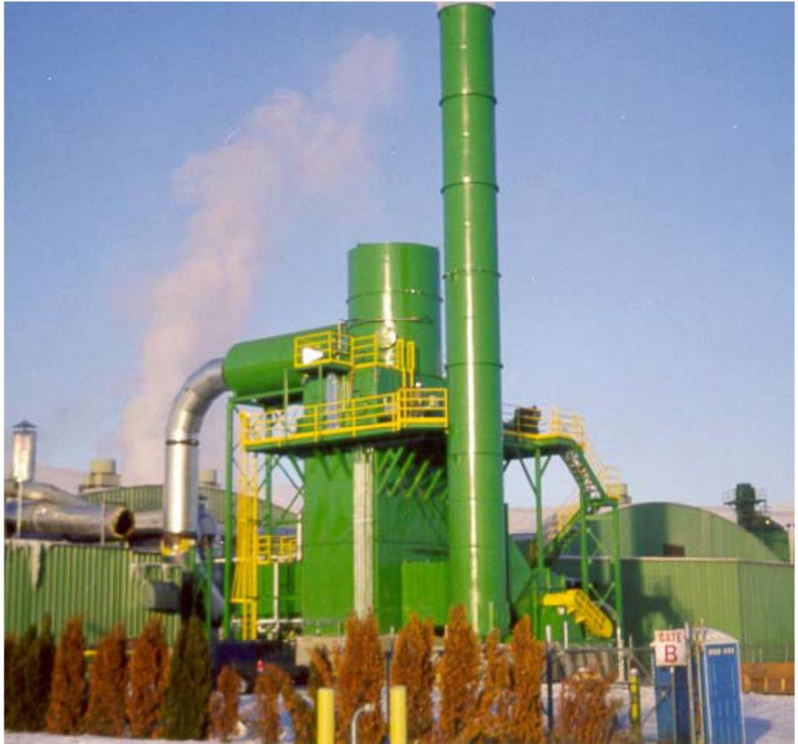
Wet ESP on a plywood veneer dryer at Boise in Yakima, Wash.
